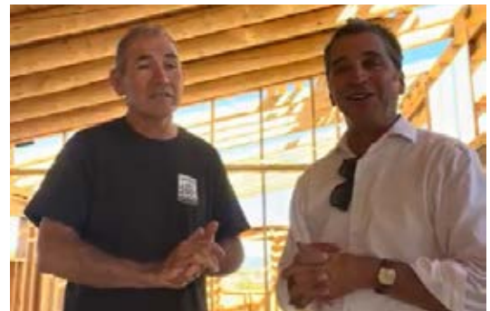
View of the newly installed vigas in a video tour with Mike and Miles
